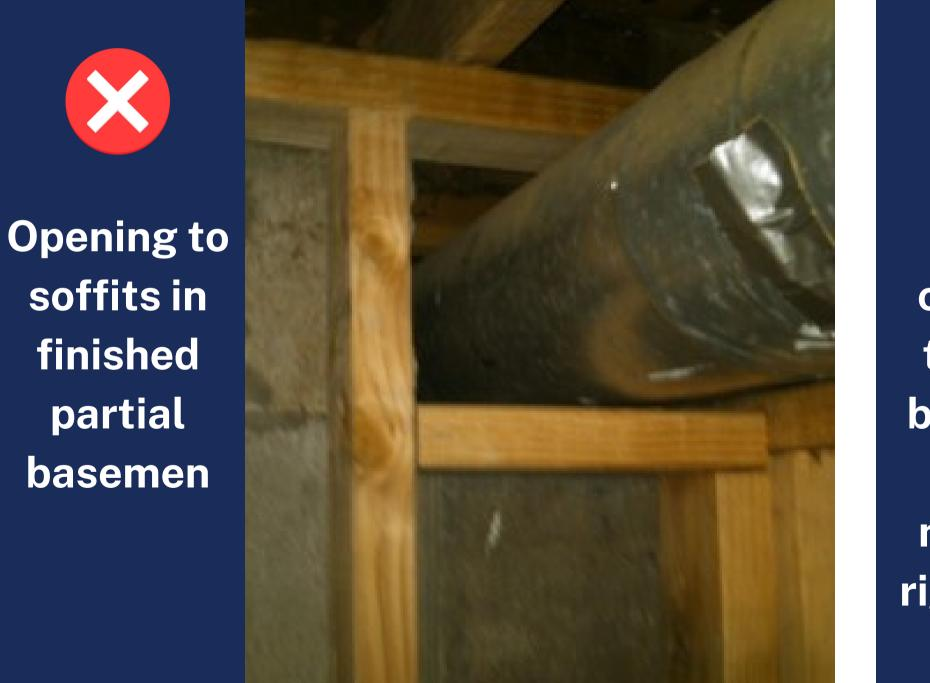
Seal chase at thermal boundary with metal or rigid foam
