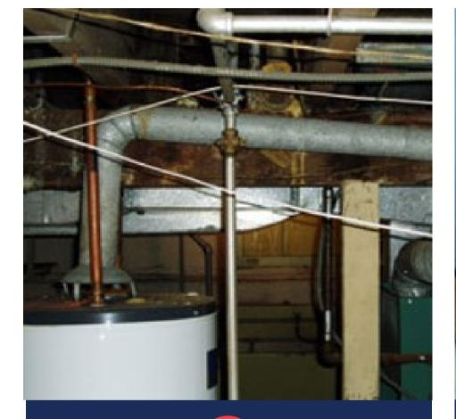
Vent damaged, sloped down, or rusted out
