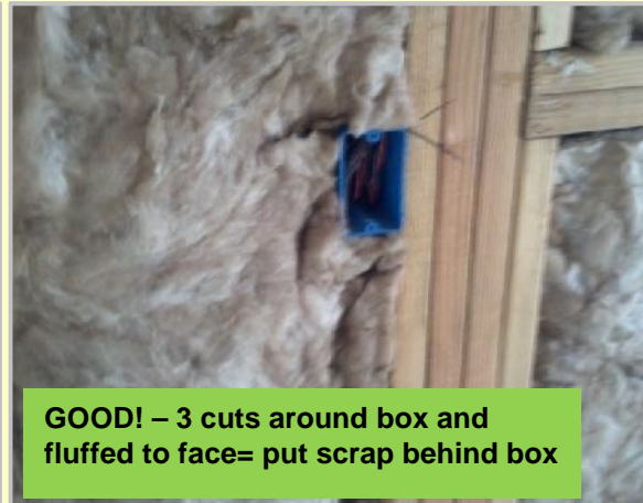
GOOD! – Fluffed to face of stud
