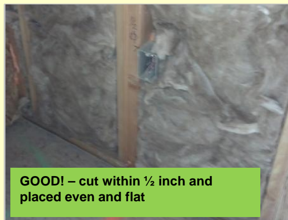
GOOD! – 3 cuts around box and fluffed to face= put scrap behind box
